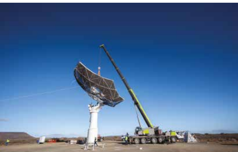
The "big lift" of the main reflector onto the telescope pedestal was performed by a team from the SKAO, SARAO and China's CETC54. Credit: SKAO
