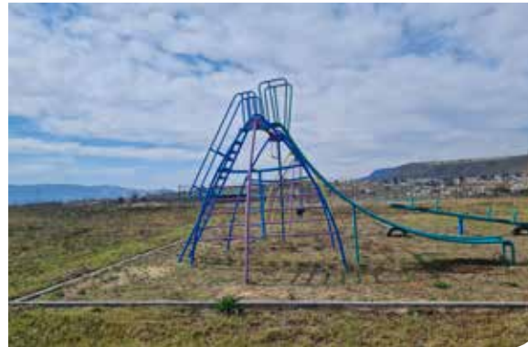
Construction of outdoor gyms and children's play parks
