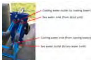
Desalination unit piping
