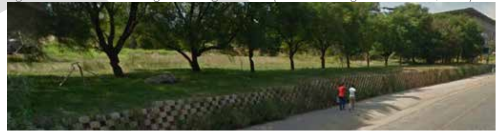
Figure 8: Pedestrian Walkway along the M5 between Zandspruit and Honeydew (Source: Google Street View, 2017)
