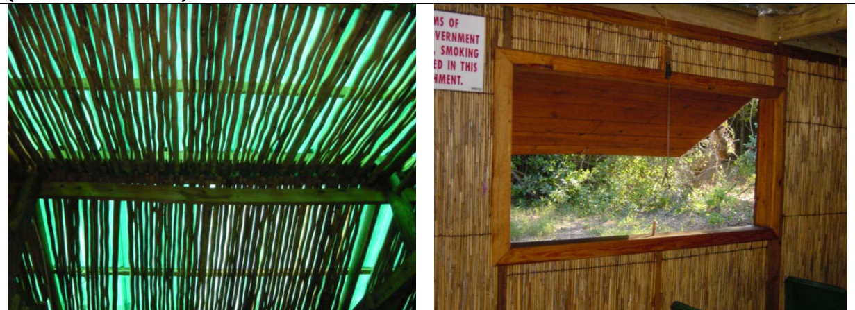
Plate 2: Responsible use of natural lighting and ventilation in building design at Coral Divers, Sodwana Bay ( www.coraldivers.co.za )
