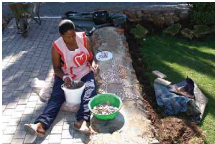
Nellie working on the wall
