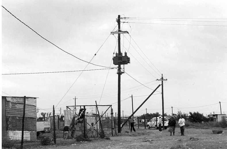
Figure 2: Bare MV and abc LV overhead conductors
