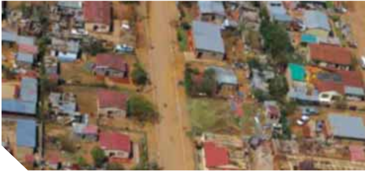
Figure 19: Damage caused by the Matlosana Wind Storm
