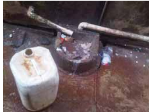
Broken & blocked drain, Thohoyandou private accommodation
