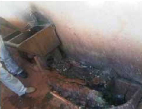
Trough where washing, laundry and cooking takes place, Thohoyandou private accommodation
