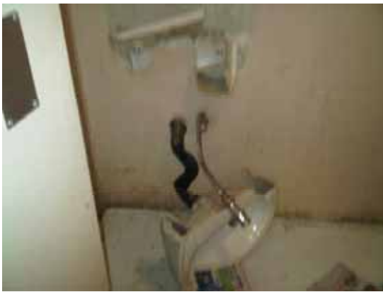
Broken basin, UL Turfloop
