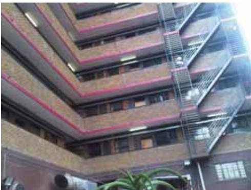
Exterior view of converted block of flats, South Point
