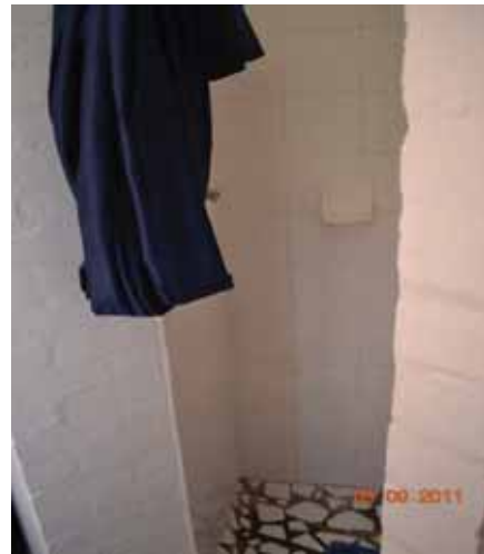
Cullen Bowles residence: ablution area
