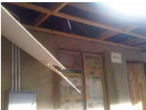
Collapsing ceiling, Thohoyandou private accommodation
