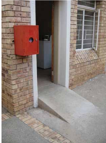
Ramp to laundry, NWU Mafikeng
