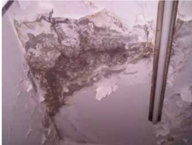
Ceiling of food production kitchen, Lonsdale, MUT
