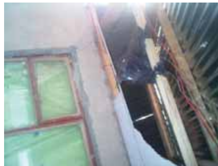
Exposed wiring, broken coverplate, Thohoyandou private accommodation
