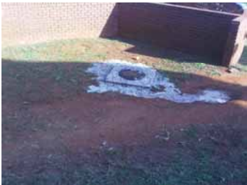
Overflowing sewerage manhole outside residence, UV
