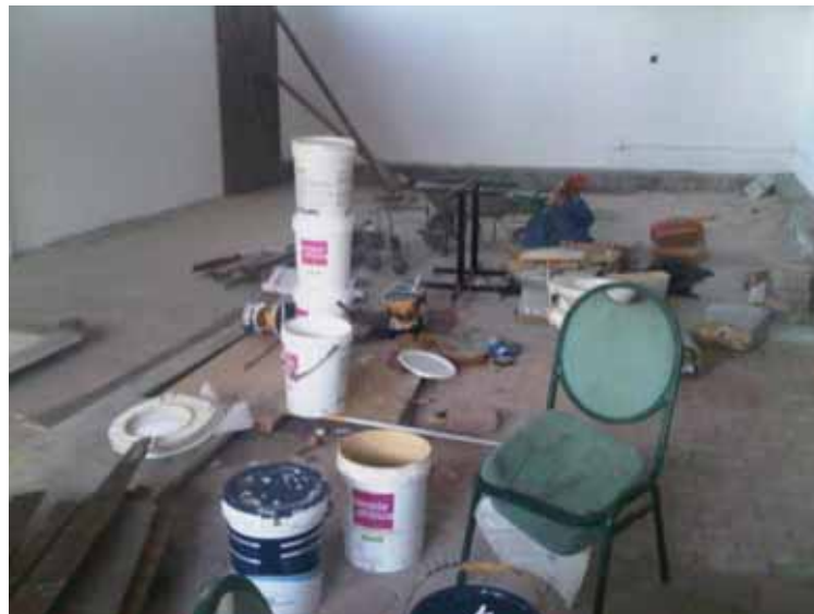
Common room left unfinished by landlord, Sikelela, CPUT
