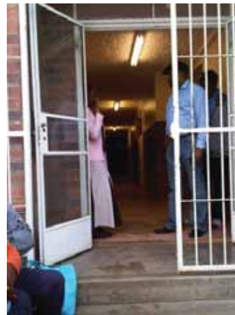
Broken and bypassed access to female residence, UFH
