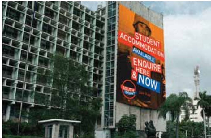
External view, South Point
