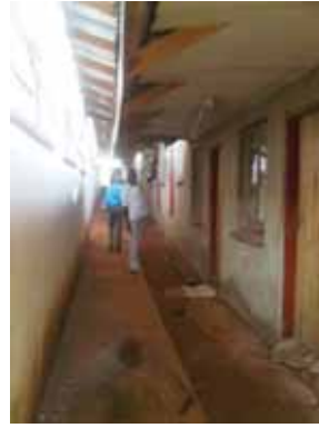
Collapsing ceiling which allows roofway access to rooms, Thohoyandou private accommodation
