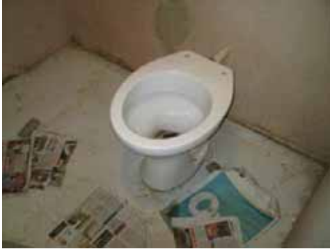
Broken toilet, UL Turfloop
