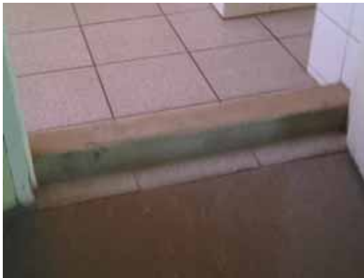
Step blocking access to bathroom for students with disabilities, CUT
