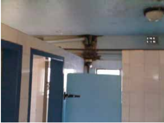
Leaking pipe in ablution area, UL Turfloop
