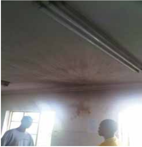
Burn marks on wall and ceiling caused by oil fire, WSU
