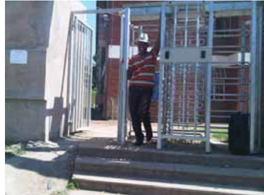
Broken access control and unlocked security gate, DUT Midlands
