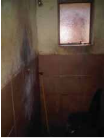
Shower, Thohoyandou private accommodation
