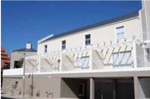
Entrance to underground parking, City Edge
