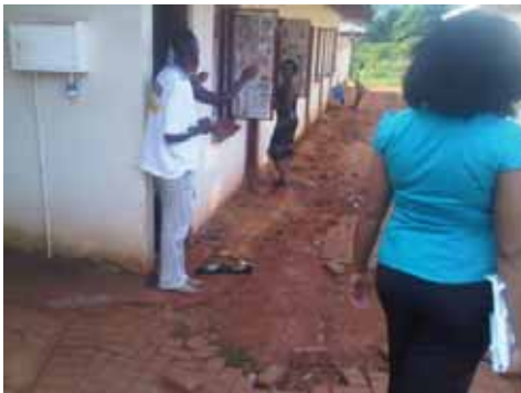
Unpaved walkway between blocks, Thohoyandou private accommodation
