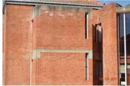
Exterior of Cullen Bowles residence (water damage)
