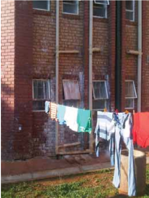
Sewerage flowing down exterior of building, UV
