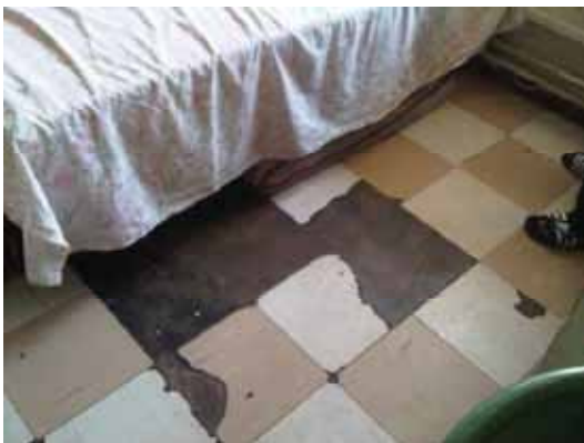
Floor of student room, UL Turfloop
