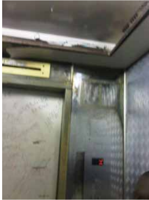
Dilapidated lift at Lonsdale, MUT
