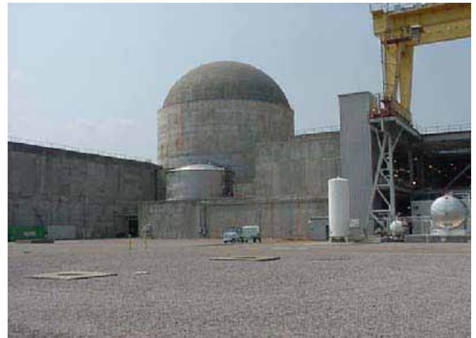
Fig 9: The dome-shaped containment building at the Nuclear Power Plant
