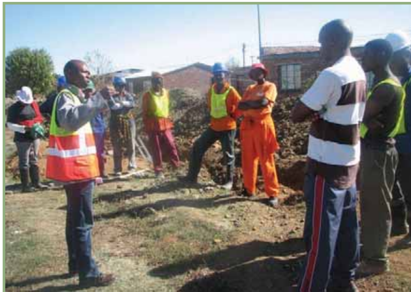
Paul Jeli explaining to workers why their construction site has to be shut down.
