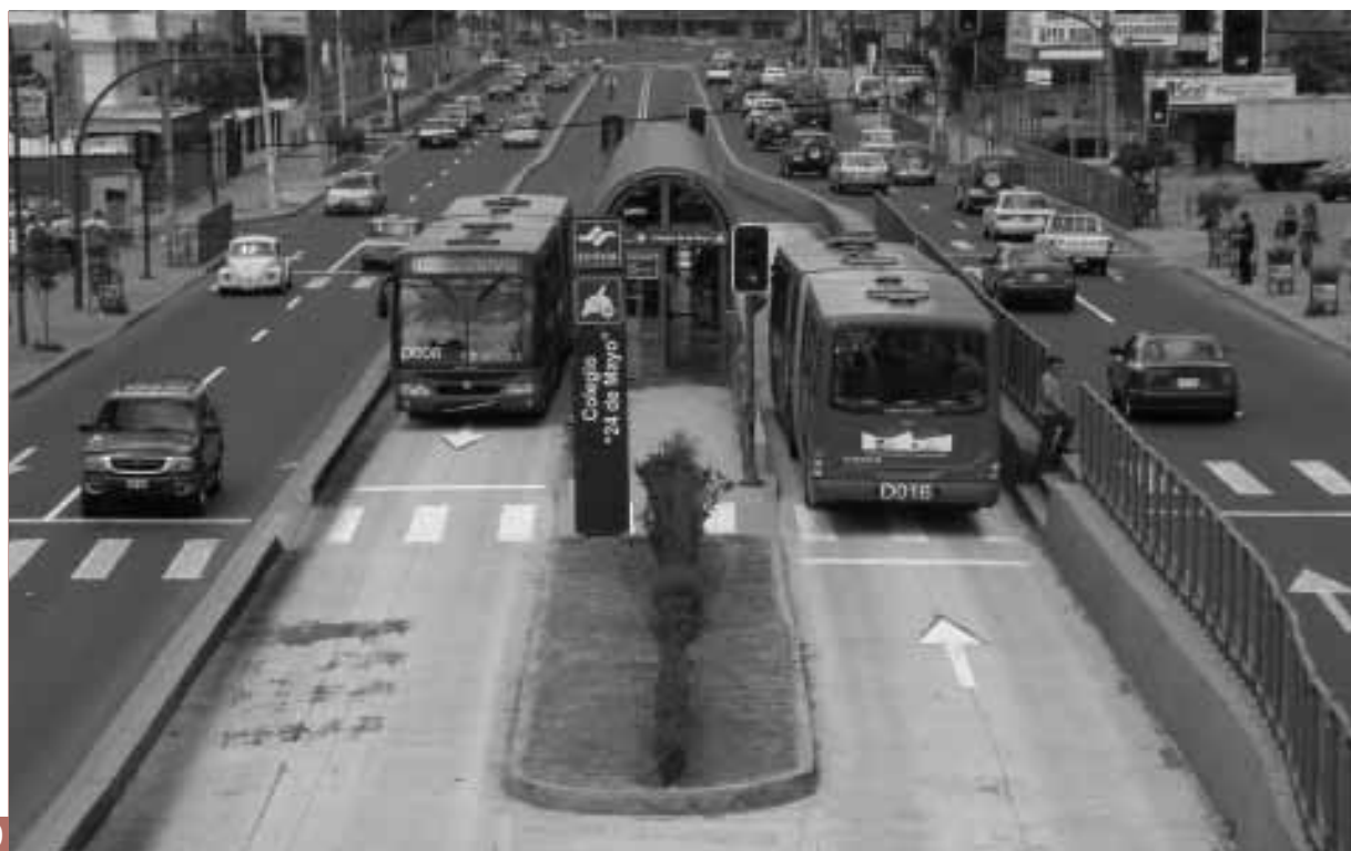
Figure 39: Transmilenio system showing median lane and station
