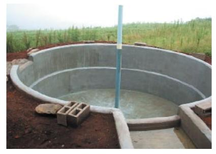
Figure 3: Typical 30 m<sup>3</sup> rainwater tank
