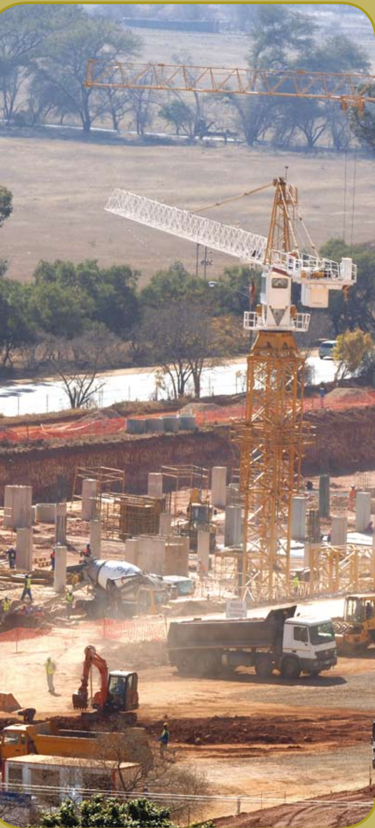
The construction site for the new DFA Head Office
