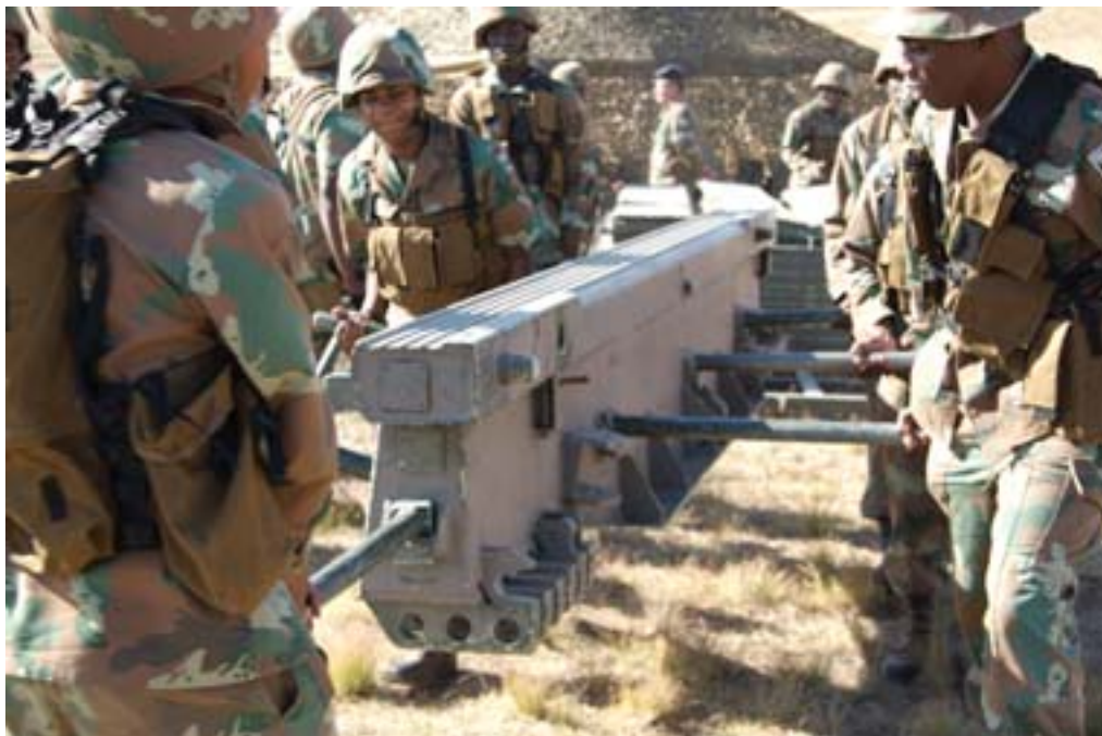
Field engineers erecting a Medium Girder Bridge (MGB) during field operations.
