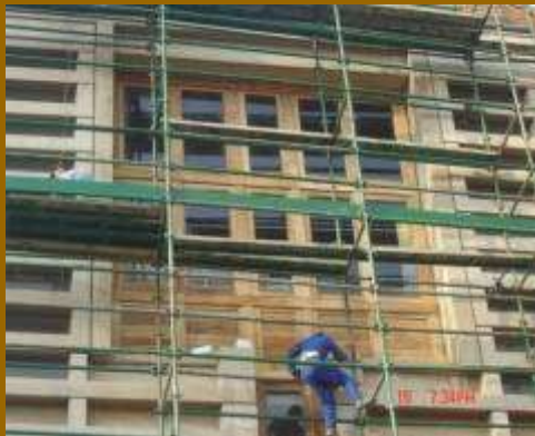
Treatment of External Timber
