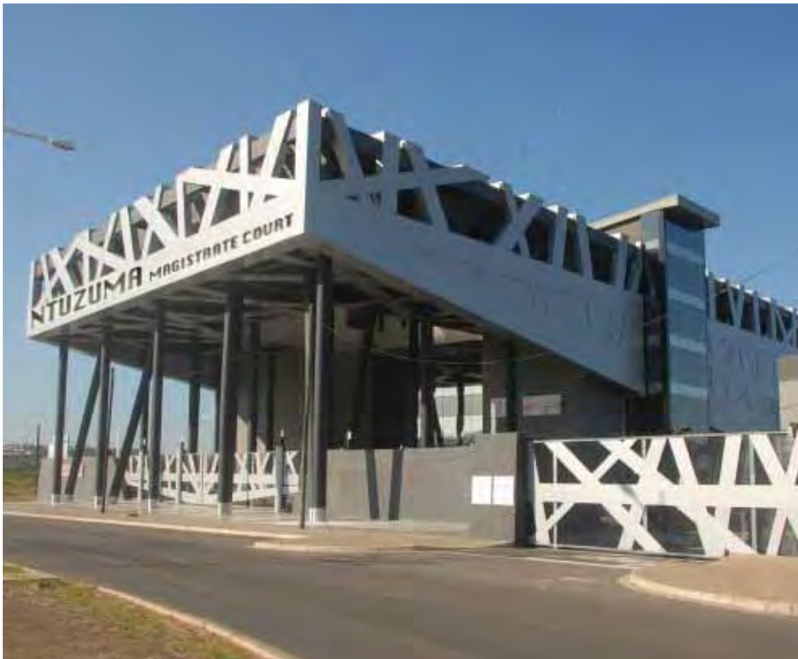
The new Ntuzuma Magistrate Court in KwaZulu-Natal is a multi-storey facility to improve access to justice to the community, this facility will be officially opened during 2012/13.
