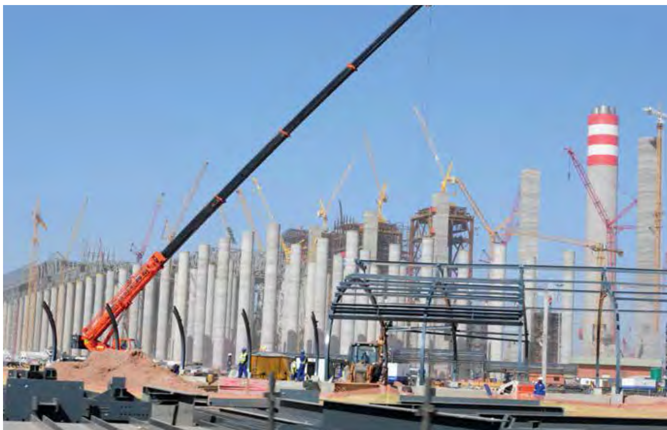
Construction of Medupi power station
