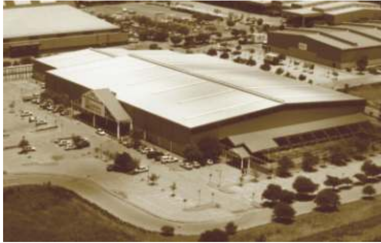
Data processing centre
