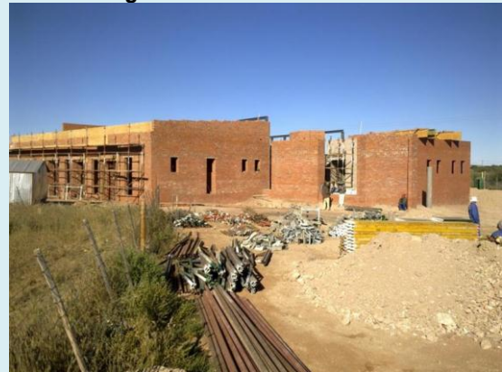
North facing view
