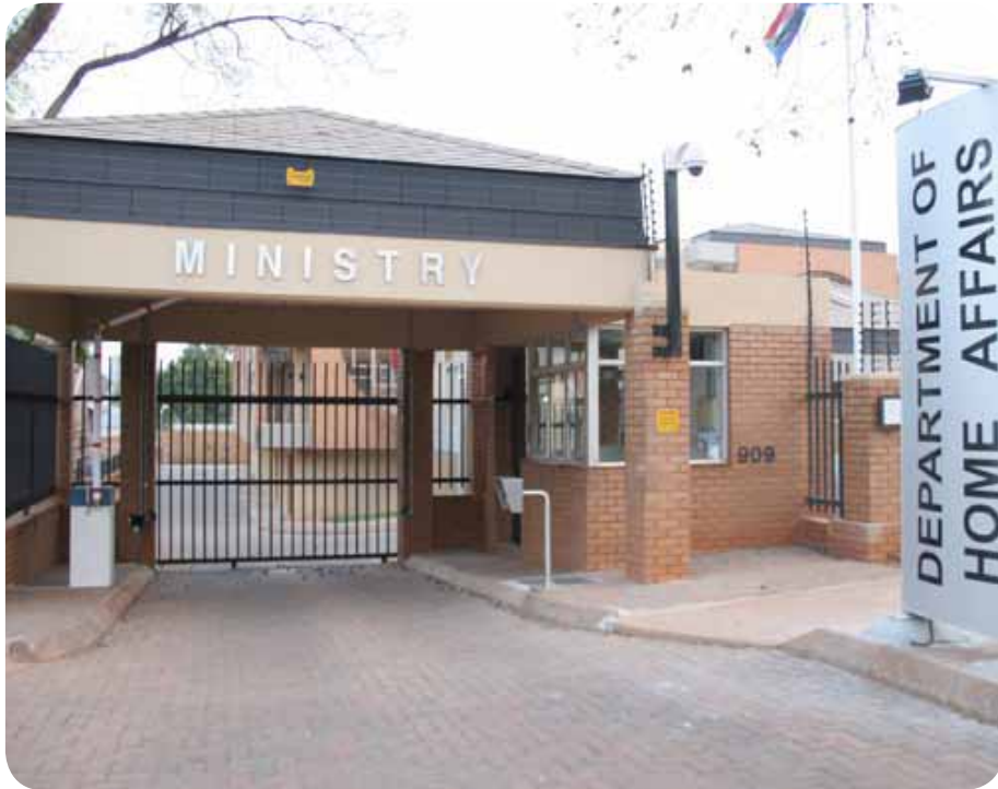
The new Ministerial offices of the Department in Acardia, Tshwane are part of the Repair and Maintenance Programme (RAMP) project of the Department of Public Works
