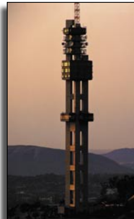
Telkom tower in Pretoria.
