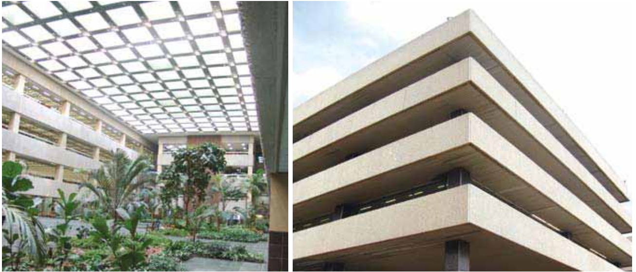
SARS Large Business Office at Megawatt Park
