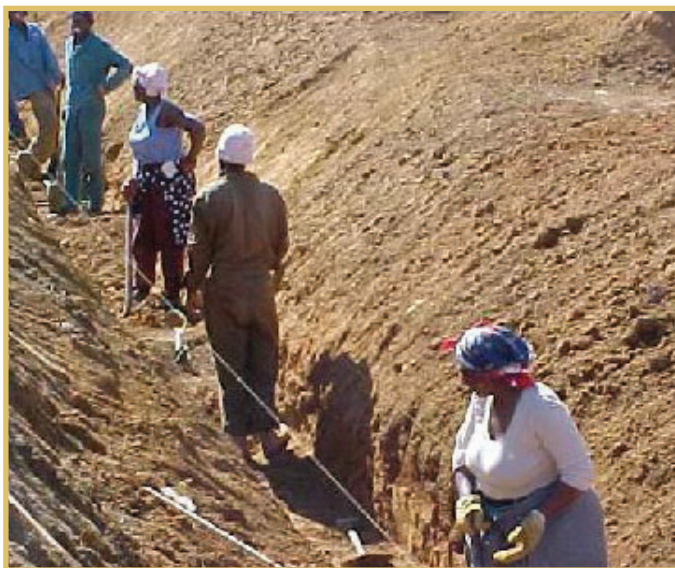
Gauteng: Johannesburg Metro, Orange Farm: Bulk Stormwater drainage
