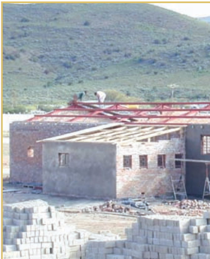
Western Cape: Prince Albert Municipality, Klaarstroom North: Waste disposal site.
