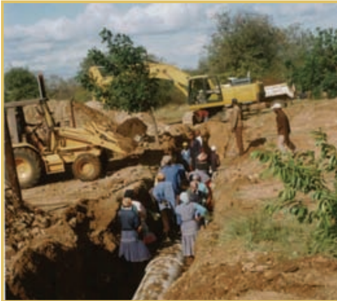
Limpopo: Mopani District Municipality, Senwamokgope, Lemando Kop, Sephukudje: Water Upgrading Project
